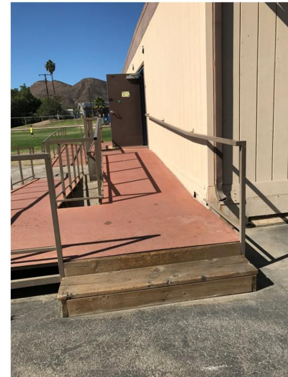
Photo 2- The building step is unsafe. Handrail is required
