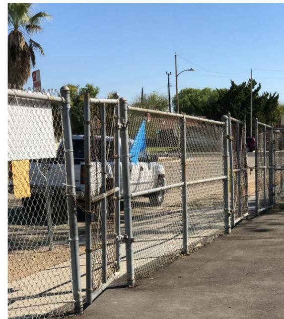
Photo 4- Chain-link fence deteriorating in places.
